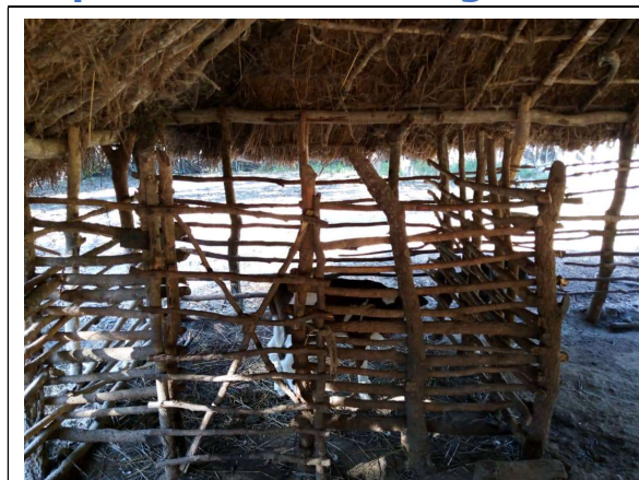
Thatched roof and walls from local poles. Shade, ventilation and protection from rain.
