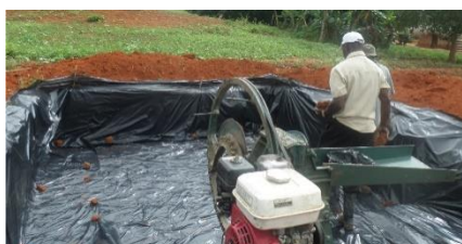
Pit lined with plastic to prevent water entering
