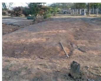
Pit closed, covered with plastic and a soil heap to let water run off
