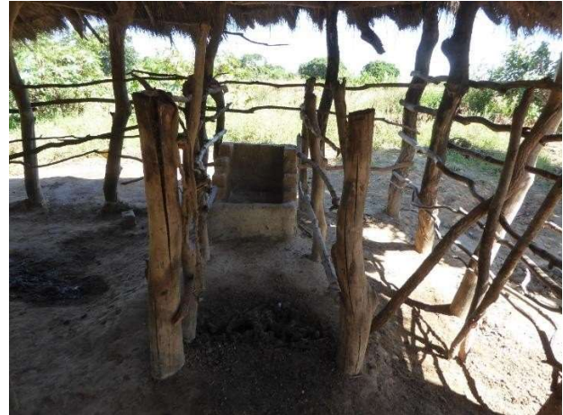
Parlour with feeding trough, thatch roof and floor sloping away to allow easy draining.
