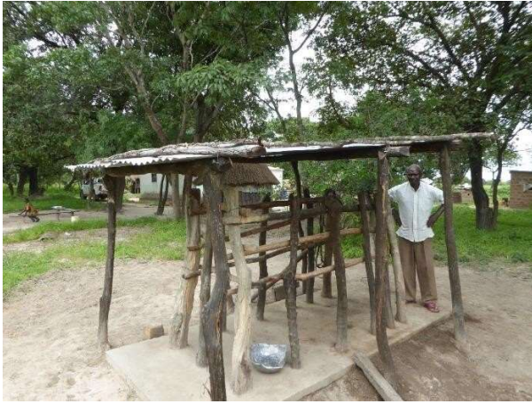
Parlour with sloping roof and raised concrete floor to allow water to drain away.
